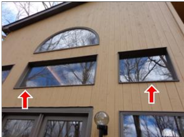
2.0 Picture 1 these windows both sides
