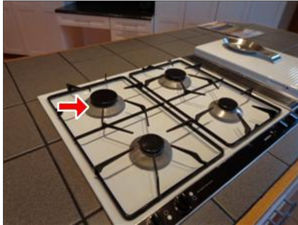
10.1 Picture 1 not lighting
