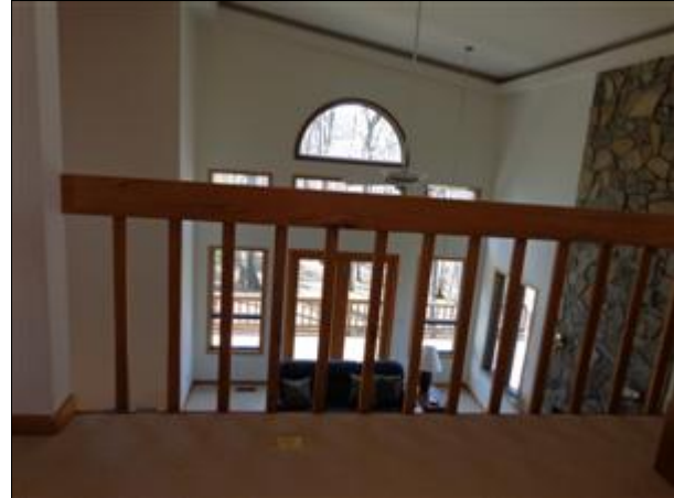
4.3 Picture 2 upper railings
