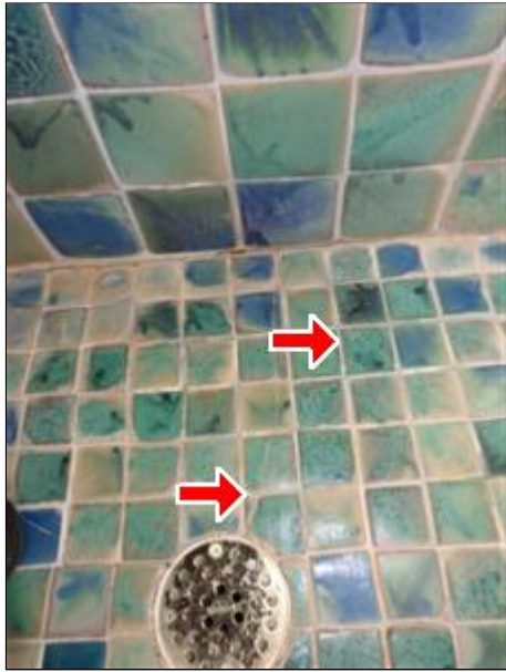
6.6 Picture 4 crack here
