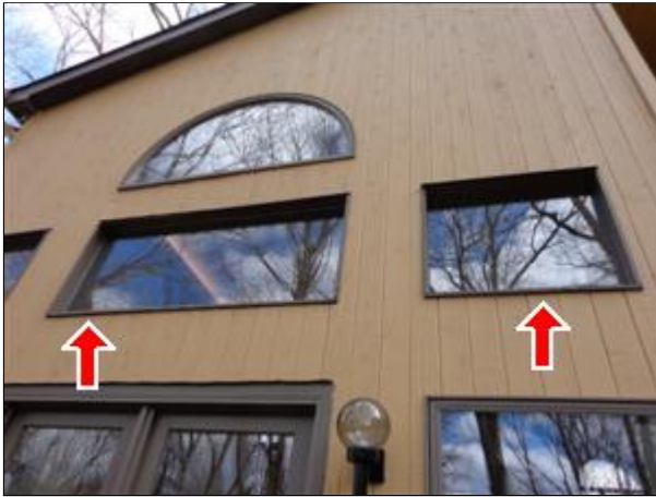
2.0 Picture 1 these windows both sides
